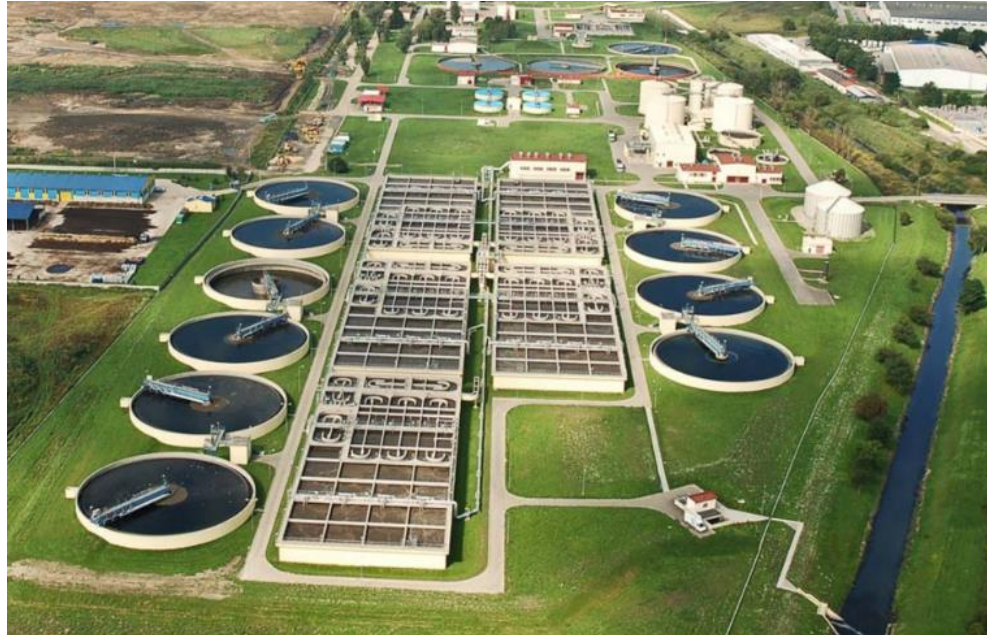
Fig. 26. Płaszów Sewage Treatment Plant in Kraków – reactor and settlers in the first plan
