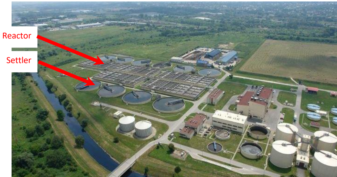
Fig. 28. Aerial photography of the Płaszów WWTP with reactor 4
